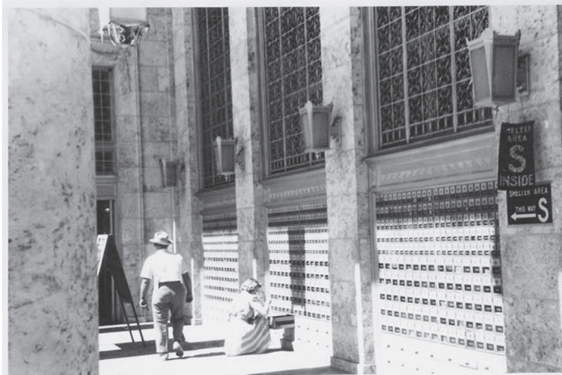
Original Post Office Boxes from the 1930s
